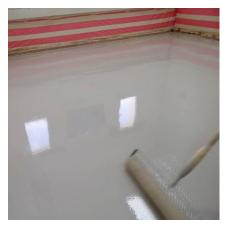
According to the manufacturer's instructions, Ucrete is mixed with a mechanical mixer. The mixed material is then poured onto the substrate and spread evenly using a pin screed rack to achieve a uniform thickness. To release any air that may have been trapped during the mixing process, the freshly applied Ucrete is then rolled with a spiked roller. This step helps to eliminate air pockets, ensure proper adhesion, and provide a smooth and even surface for the final cured screed.
