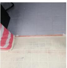
In order to prevent the polyurethane screed from debonding from the concrete substrate, grooves are cut into the concrete to provide an anchor for the Ucrete MF.
