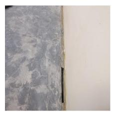
Once the vinyl flooring was removed, it was crucial to eliminate any remaining residue, especially the glue that was used to secure the vinyl tiles. The surface was then ground, cracks were filled, and thoroughly cleaned in preparation for the final top layer of polyurethane screed, Ucrete MF. As per the instructions of technical personnel from Master Builders Solutions, grooves were incorporated into the flooring to meet the product requirements.
