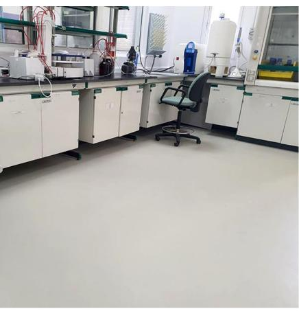
The flooring system applied in the project consisted of Ucrete MF, which was applied at a thickness of 4 mm in the corridors, Ucrete HF 60 RT at 6 mm thickness in labs and chemical stores, and Ucrete RG for coving. To ensure compliance with the manufacturer's recommended method statement, the Master Builders Solutions technical team conducted regular inspections throughout the application process. Moreover, the manufacturer provided timely supply of materials to support the project's progress.
