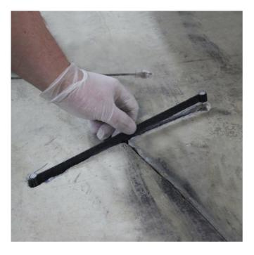
Concrete stitching is a proven and effective method for repairing concrete structures. With its speed, ease, and cost-effectiveness, it is a popular choice for many concrete repair projects, and whether using metal staples or carbon rods, this process helps to reinforce the damaged area, creating a more stable and durable structure.
