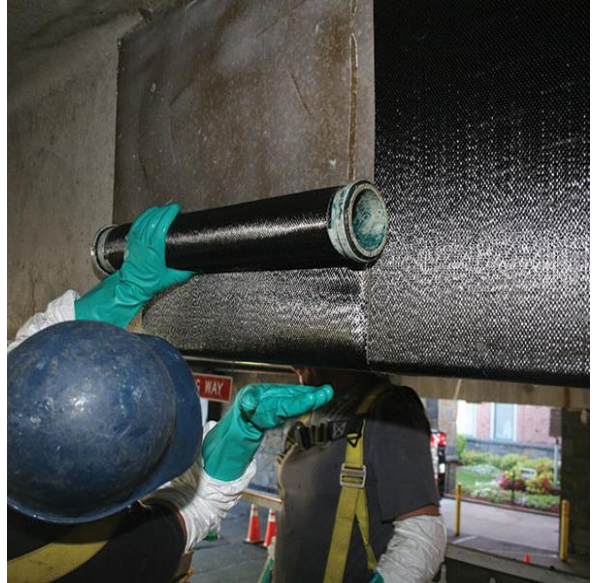
Carbon Fiber Strengthening
