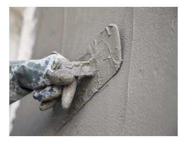
A range of advanced solutions, far beyond the simple concrete patch, was utilized to implement an effective concrete repair program. The first phase of the repair program was the cooling tower tanks. The extend of corrosion in the tanks were high, spalling had caused exposure of the reinforcement in many areas. The extend of corrosion on the tank roof slab was beyond repair and decision to demolish it and reconstruct it was taken.
