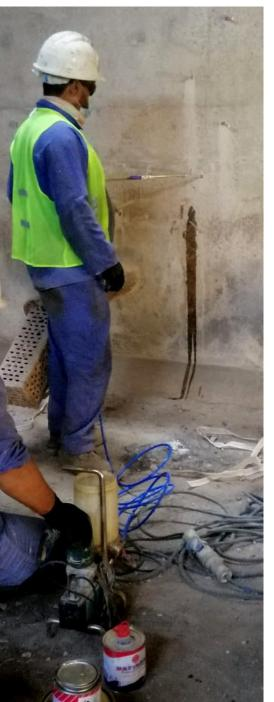
Carbonation, movement or poor construction can cause dangerous cracks in concrete structures, leading to the appearance of leaks and water penetration. Resin injection is designed to inject and seal the cracks that appear in reinforced concrete.
