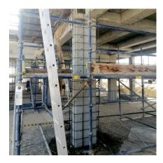
Surface preparation was done mechanically and chemically to clear the surface of pre-existing coatings, residue, surface imperfections and provide a good bond to the micro concrete. Mechanical abrasion was done with scarifier and to ensure additional bond epoxy bonding agent was used.
