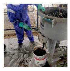
Dowell bars were anchored with epoxy anchor grout and steel reinforcement and transverse steel ties outside the perimeter of the existing structure were provided as per the structural consultant's requirement and drawings. Special care was taken in fixing the shutters as it needed to be watertight to avoid grout loss. Specialized mechanical mixers were used to mix the micro concrete. Pouring and curing the micro concrete were done as per the manufacturer's recommendations.
