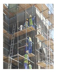
The insulation used on this project was Neopor. This is a material patented and manufactured by BASF. Composed of small grey beads of polystyrene granules containing a blowing agent, which makes it expandable, these beads are manufactured into insulation.
